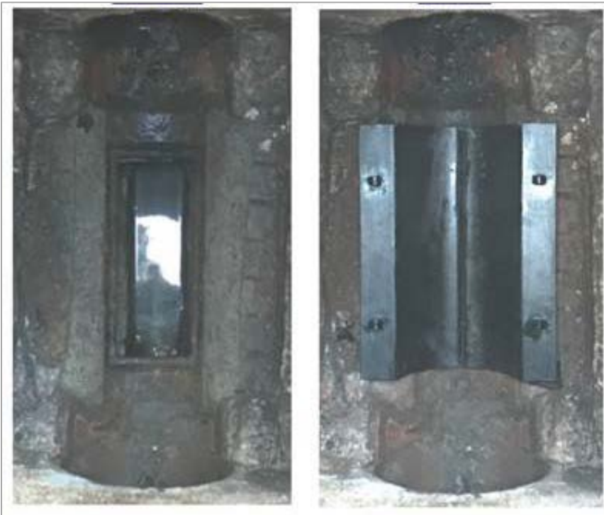
Figure 3-6. Over/Under Sewer Before/After Invert Plate Installation
