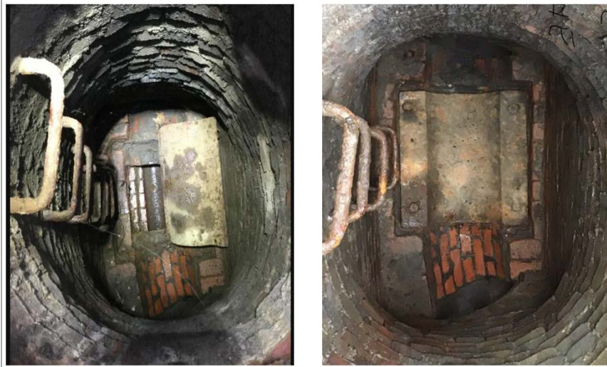
Figure 3-6. Over/Under Sewer Before/After Invert Plate Installation
