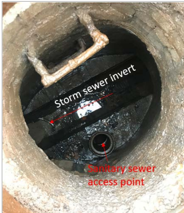
Figure 1-5. Topside Photo of Piped Access Sewer
