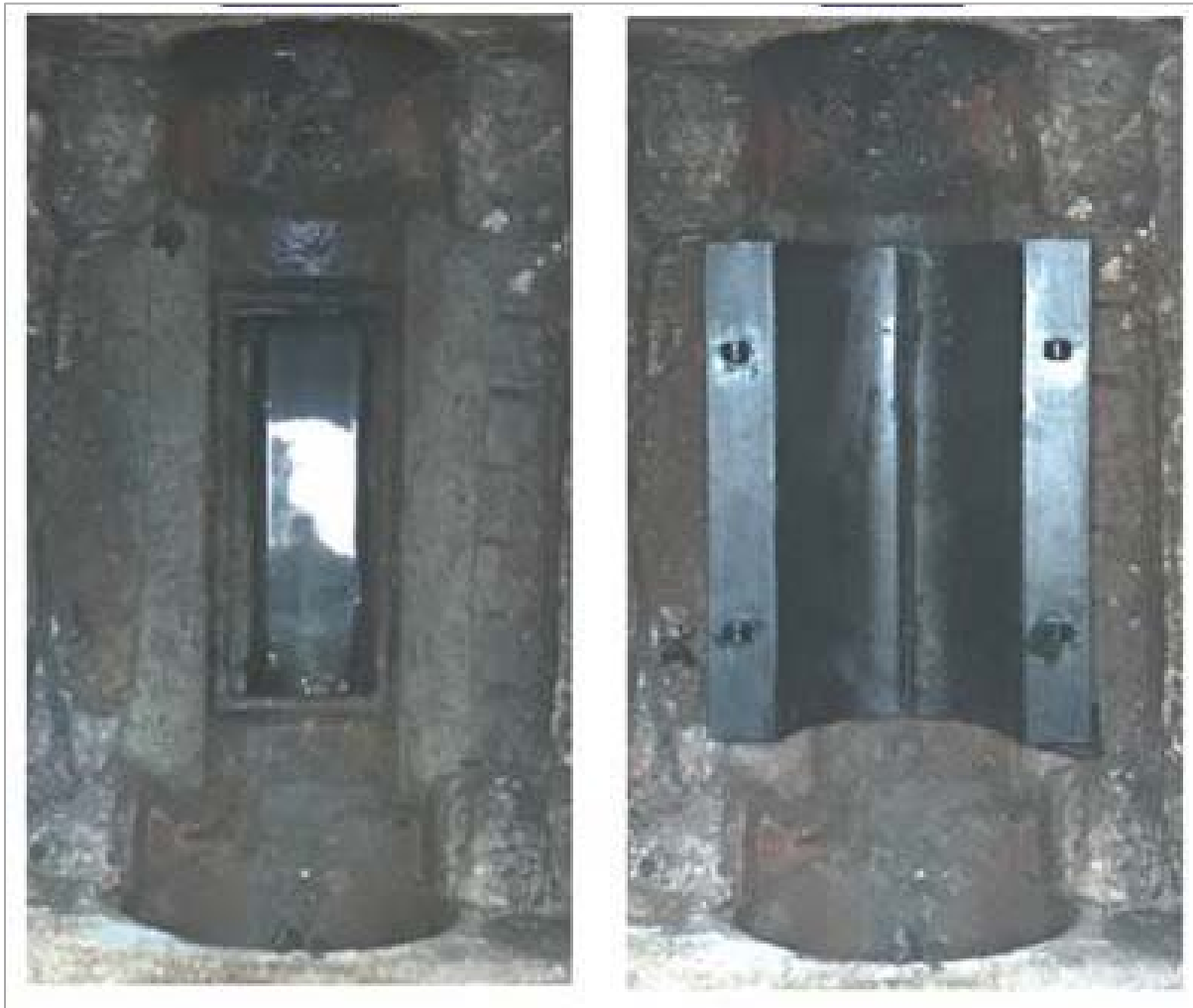
Figure 1-11. Missing and Replaced Invert Plate
