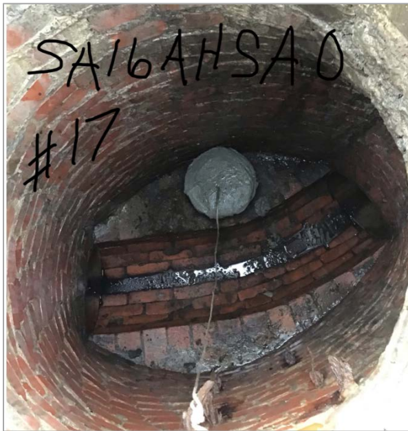
Figure 3-7. Sealed Pipe Access Manhole
