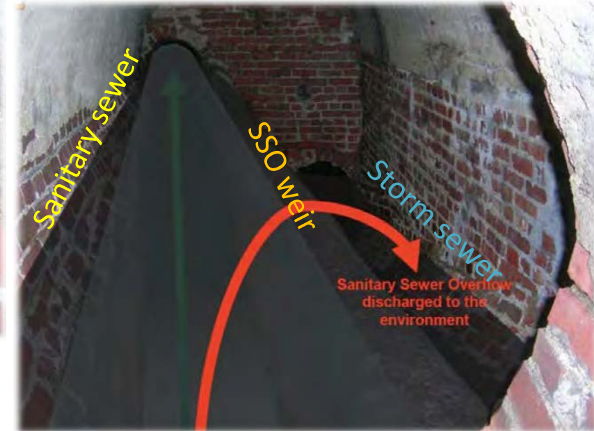
Wet weather SSO to storm sewer
