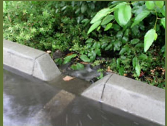
Water runoff inlet to vegetated swale
