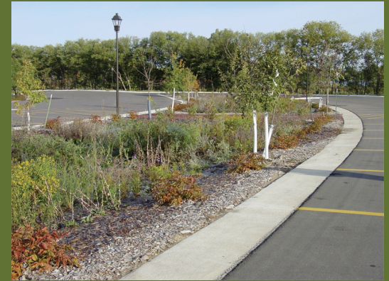
Parking lot managing runoff & stormwater with a bioswale
