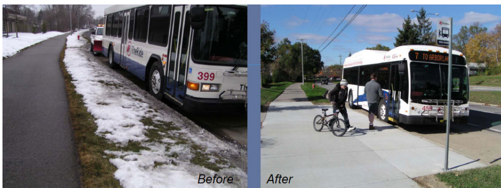
In climates with snow, ice and mud, improvements as simple as a pad to give passengers a place to board and alight the bus between the curb and the sidewalk can be a major improvement (The RIDE, Ann Arbor).
