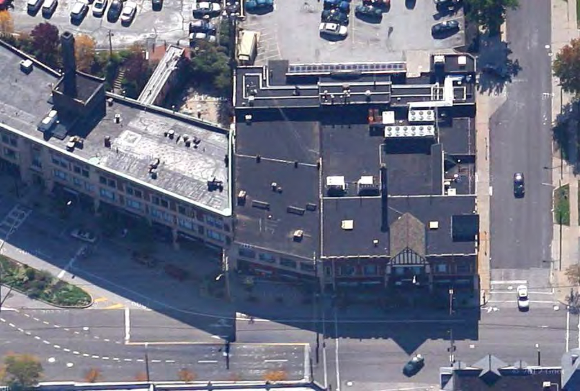
Fairmount Plaza Existing Aerial
