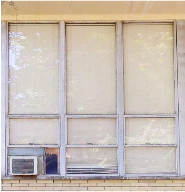
Existing anodized aluminum window
