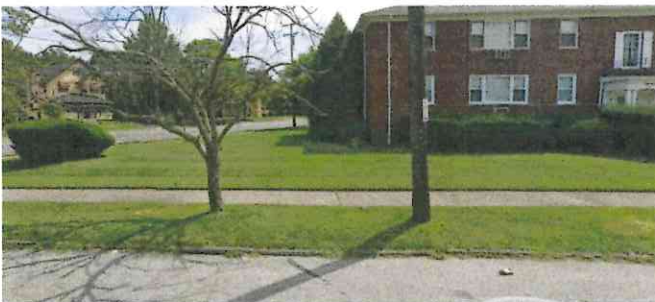
4 - NOBLE ROAD & WOODVIEW ROAD LOOKING E
