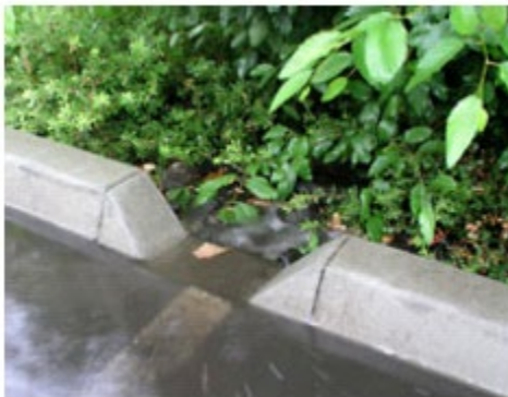
FIGURE 1166.06(b)(6): EXAMPLE OF CURB INLET
