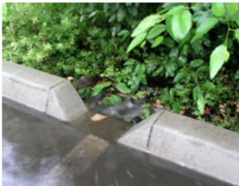
FIGURE 1166.06(b)(6): EXAMPLE OF CURB INLET
