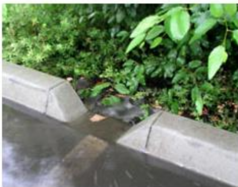
FIGURE 1166.06(b)(6): EXAMPLE OF CURB INLET
