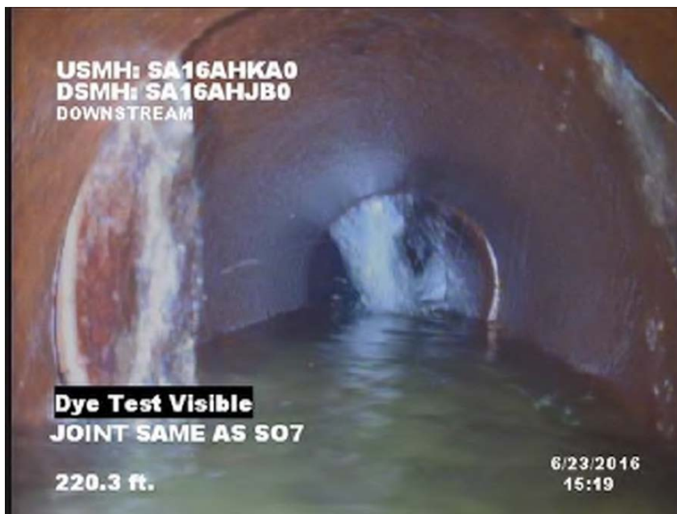
Figure 1-5. Sewer Joints Leaking During Dyed Water Testing
