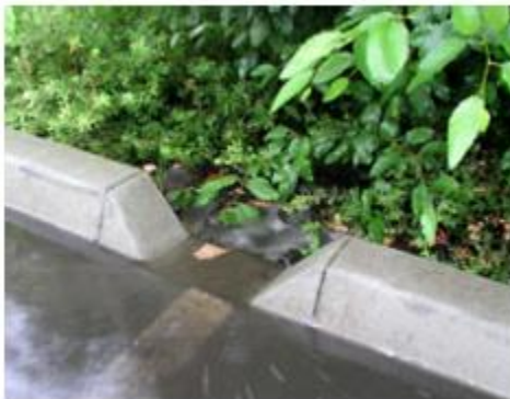
FIGURE 1166.06(b)(6): EXAMPLE OF CURB INLET
