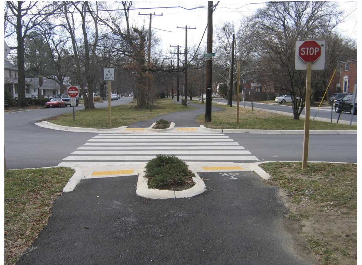
Example: Median discourages motorists while still allowing access for maintenance vehicles
